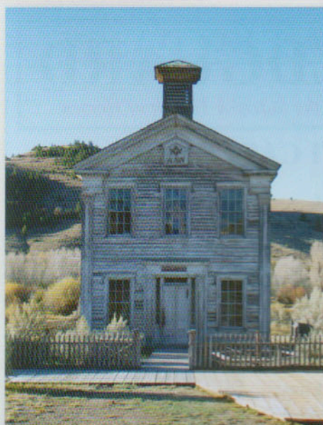
The Old School House and Masonic Lodge, Bannack
